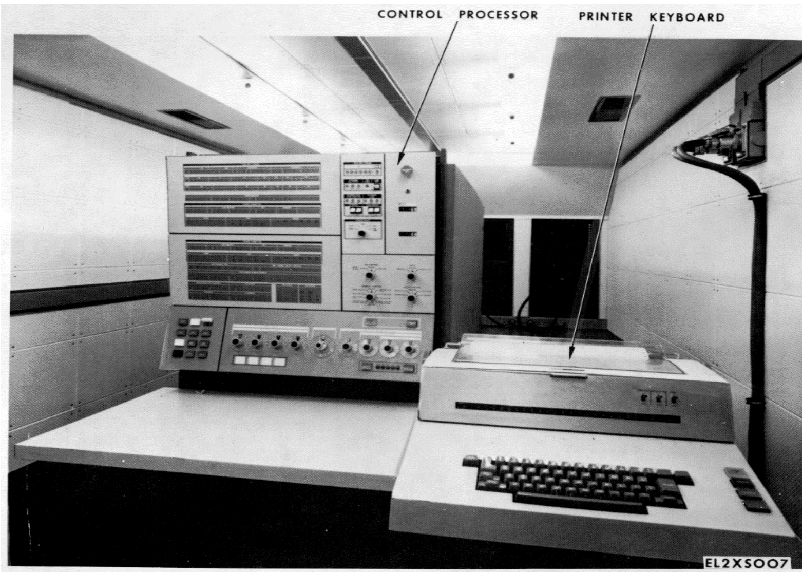
Figure 1-7. Data Analysis Central OL-88(V)1/MYK-8(V), Interior Front View.
